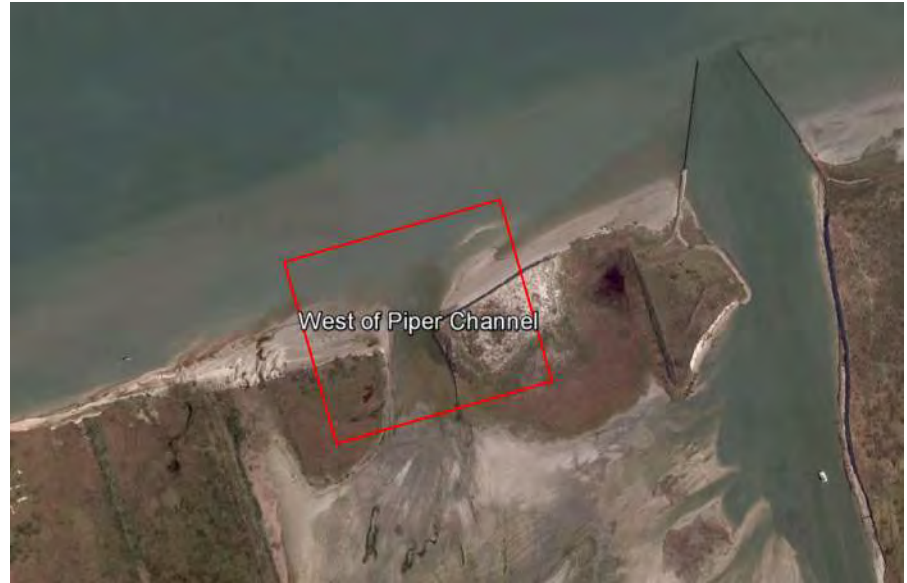
Figure 6. West of Piper Channel breach
