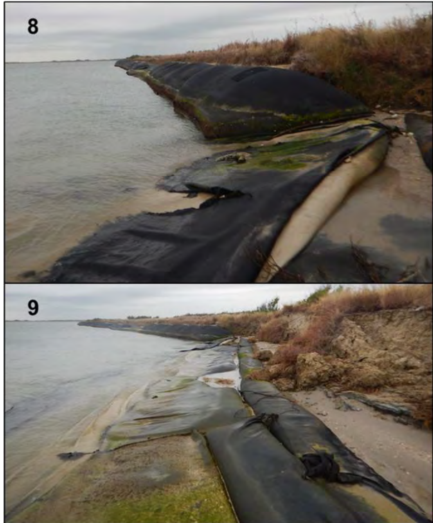
Figure 2. Harbor Island geotextile tube
